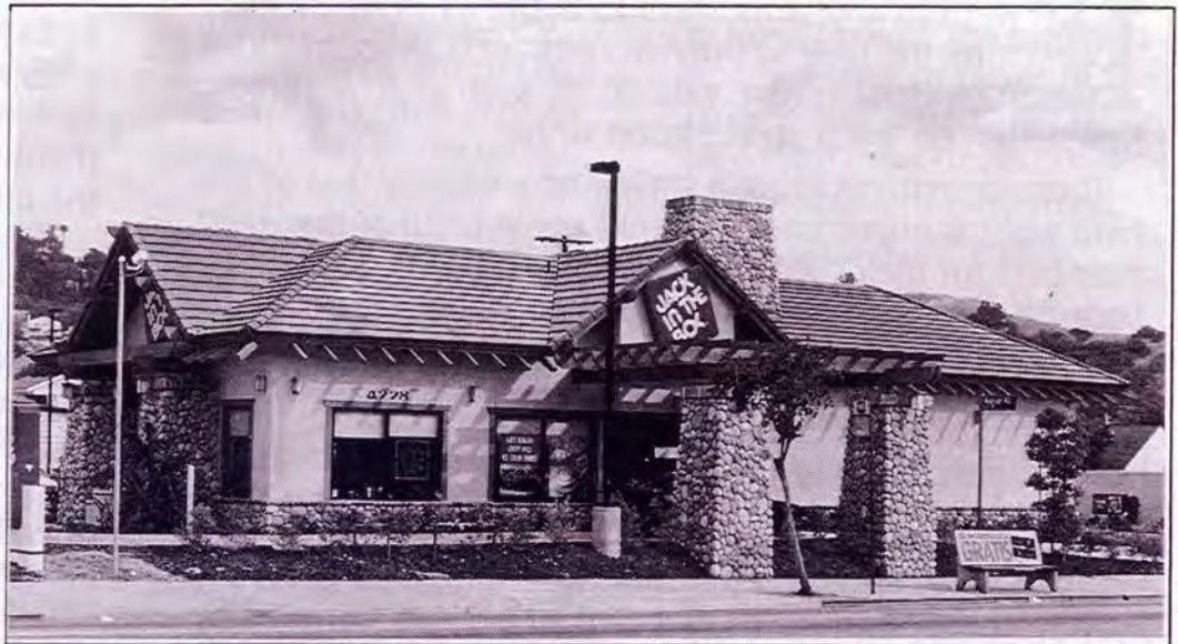
A wonderful example of new development within the Highland Park HPOZ. Thank you Jack in the Box for an eatery that also sets a design precedent!
