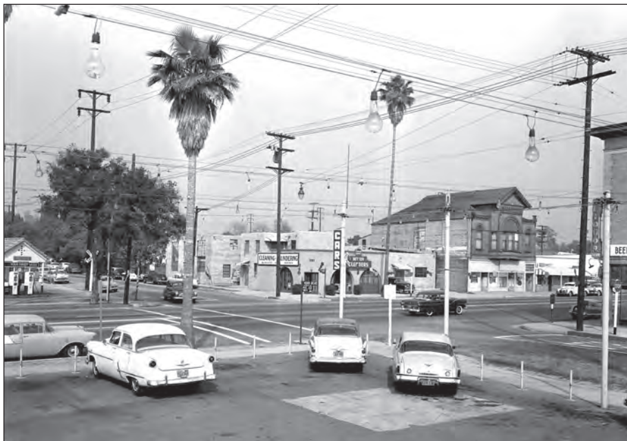
Avenue 63 & York Blvd. Photo taken in 1959 by Joe Frazier for the Northeast Newspapers shortly before the demolition of the historic Miller's Hall, which is to the right. Courtesy of Charles J. Fisher.
