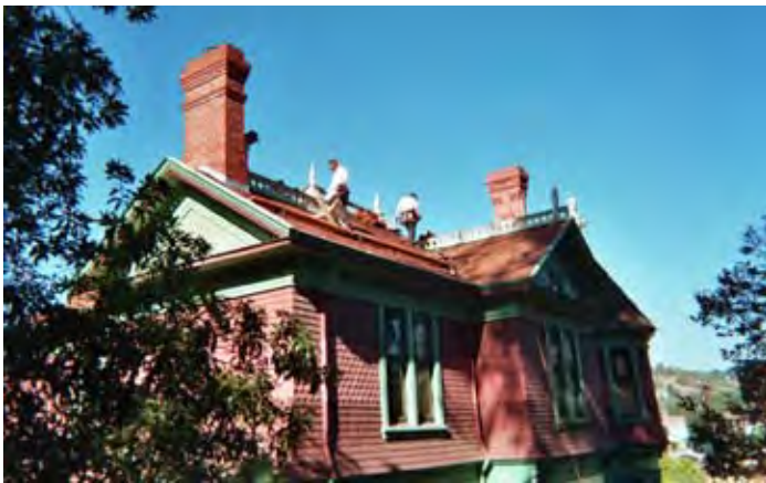
Roofers working on Hale House roof.
