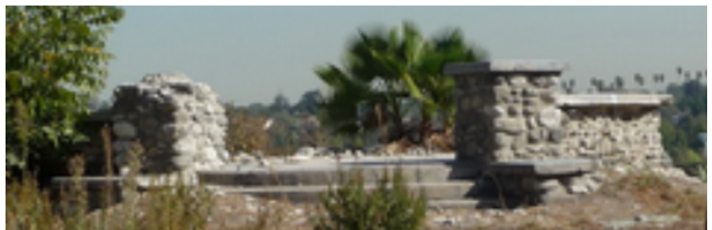
The remaining porch of the George Wilson Estate as it stands today.
