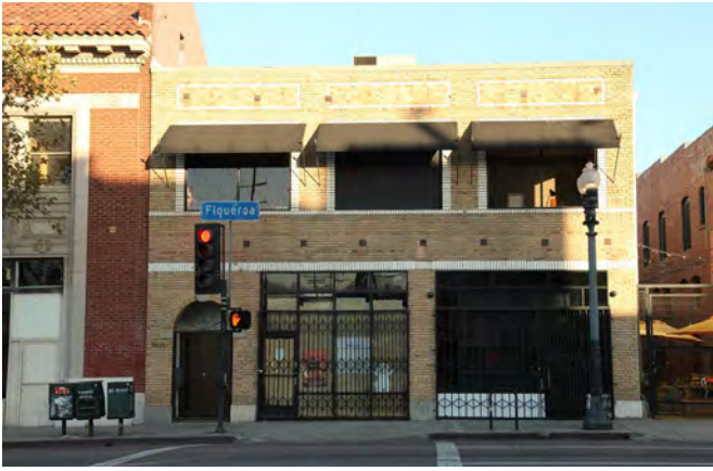
5607 Figueroa Street, former site of the Centro de Arte Publico
